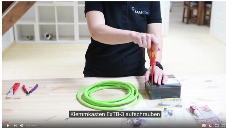
Fig. 5-5 Video Tutorial ExTB-3: Screw on the terminal box ExTB-3
